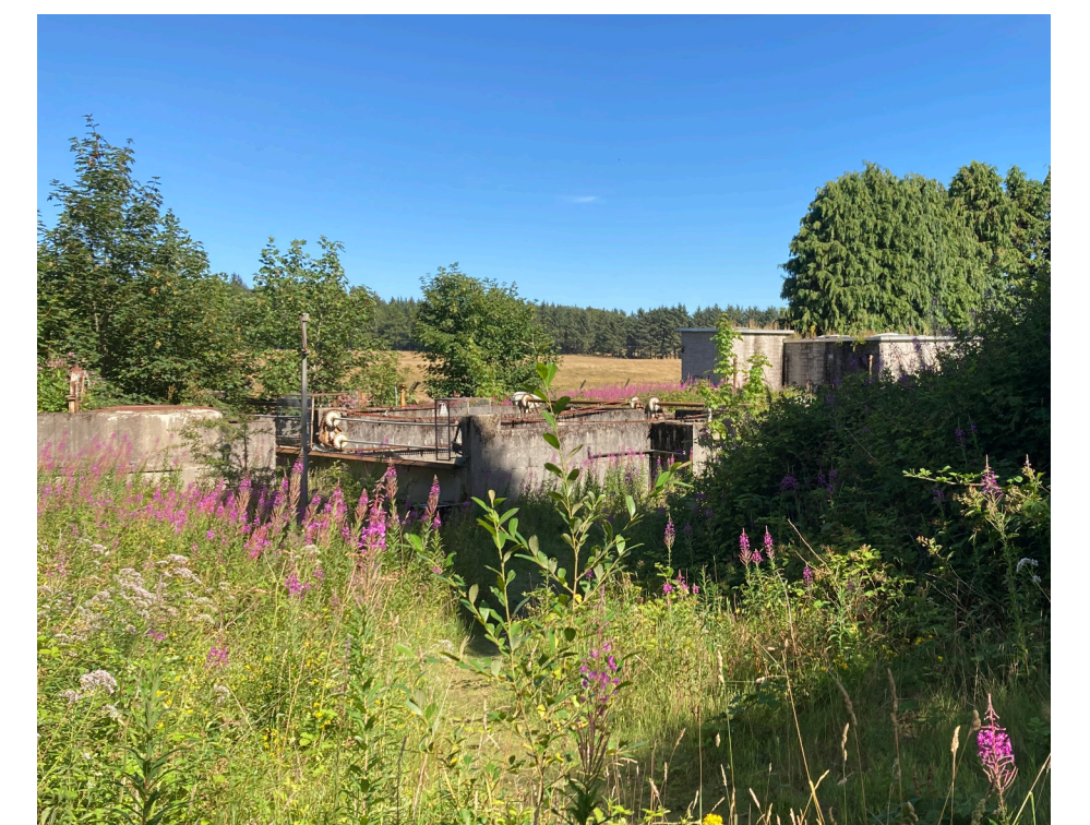
Disused Sewage works, public access discouraged.
